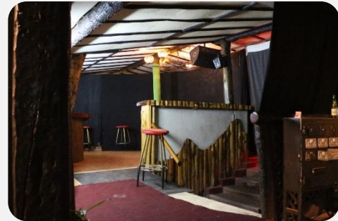
Figure 4.72 Rough, natural outer timber chunks, barks removed and varnish applied Source: Author
